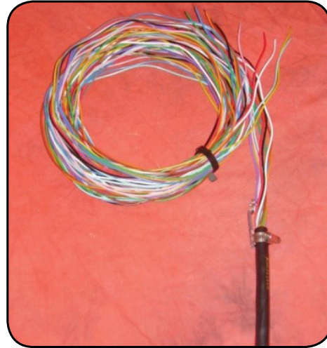
Opening End of the Cable
